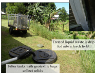
Filter tanks with geotextile bags collect solids
